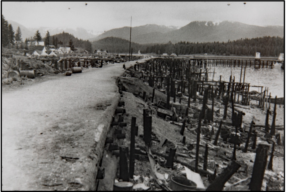
Front Street after the fire showing charred pilings of our lost waterfront homes.
