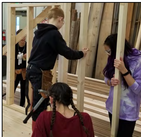
Here the framing crew is setting the walls up on the deck.
