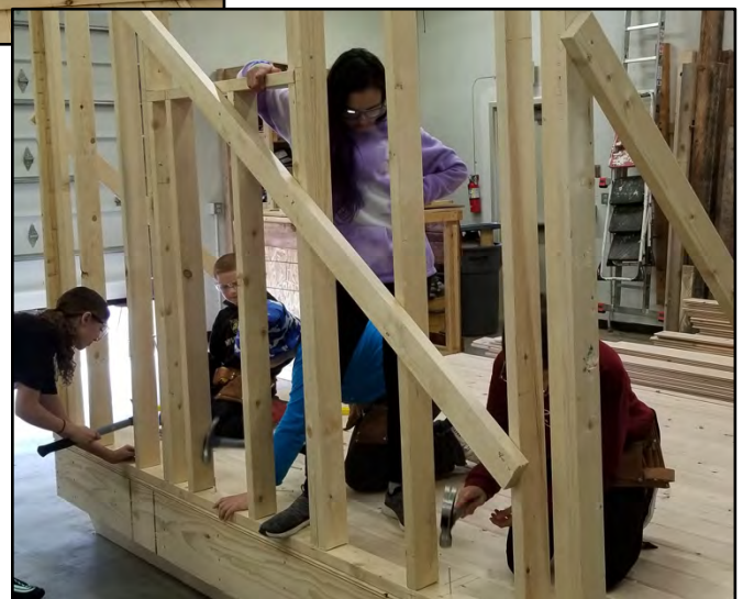
Here the framing crew is setting the walls up on the deck.
